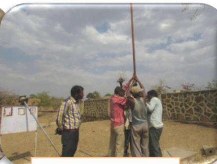
Repair of Hand Pump
